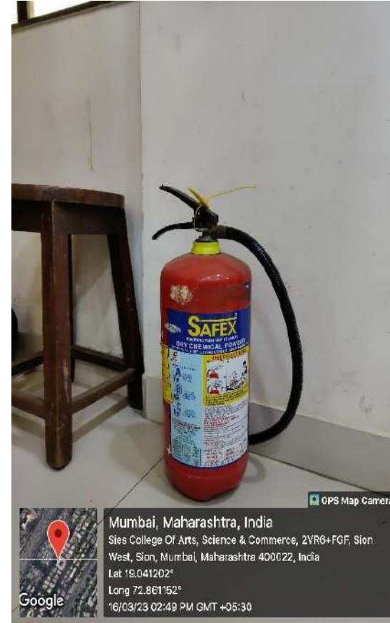
b. Fire safety
